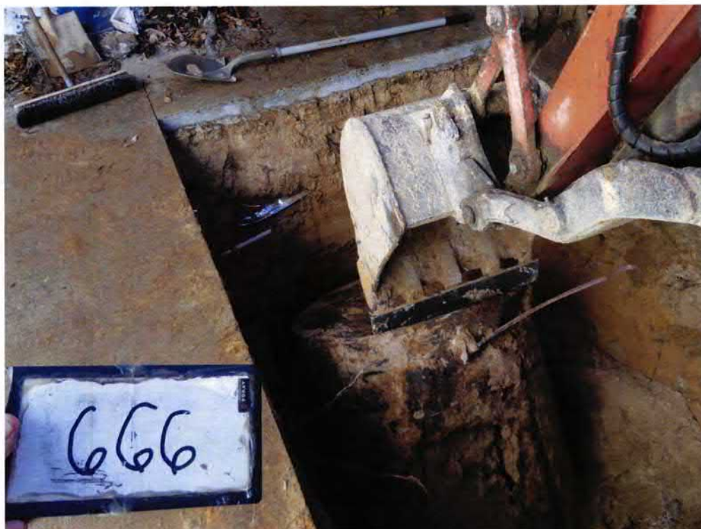
Picture 2: UST 666Camellia excavation.
